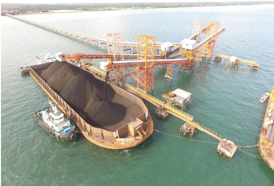
Image 1: Direct barge loading at BIB from GEAR's conveyor belts that extends 800m into the Java Sea
