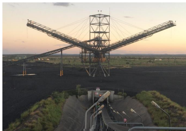
Stanmore Coal - Coal Handling Preparation Plant
